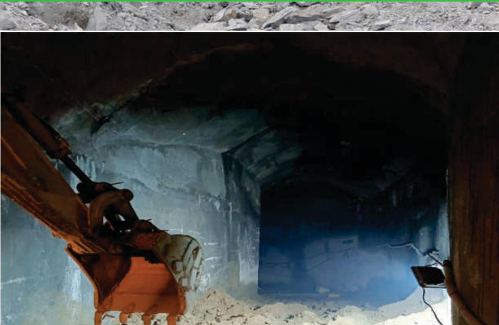
Bypass Tunnel Invert Excavation Work in Progress Shongtong Karchham HEP 450 MW
