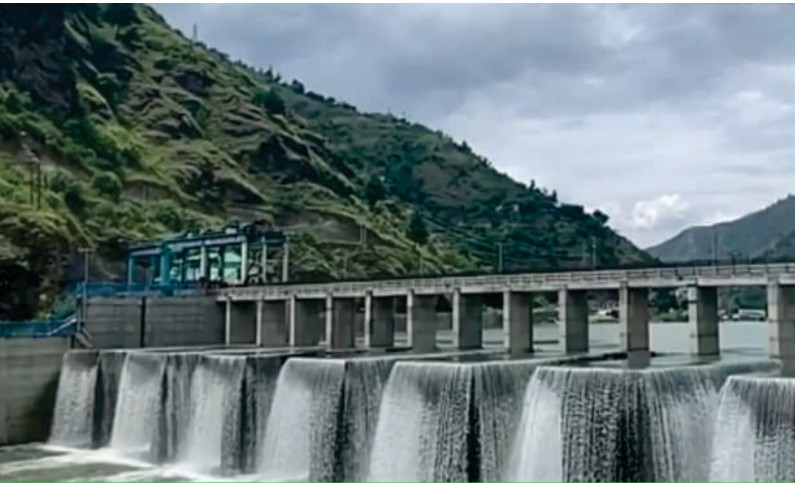
Barrage of Sawra Kuddu HEP - 111 MW
