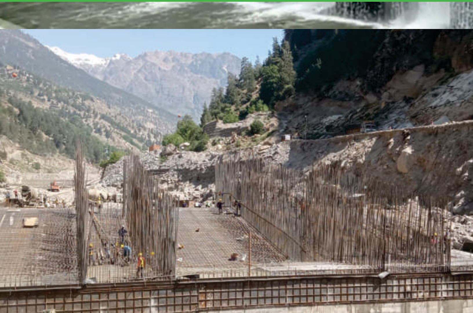
Barrage Glacis Block Concreting & Reinforcement Works - Shongtong Karcham HEP 450MW
