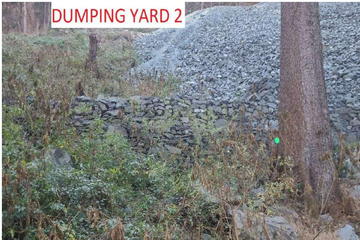
Fig No. 2 – Dumping Site2
