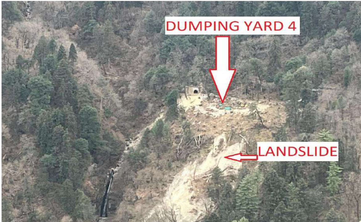
Fig No. 3 – Dumping Site4
